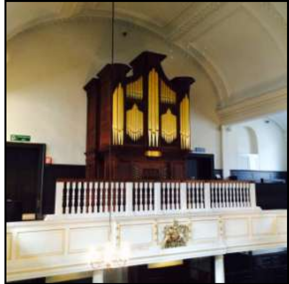
Newly installed balustrade
